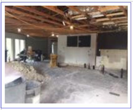
Speaking of safety, everyone on site needed ear protection early in the week with lots of hammering and cement saws. All the tile in the entrance way has been removed and they have cut through the foundation to access the sewer lines. As you can see in the photos, all the supporting plumbing for the bathrooms is now complete.
